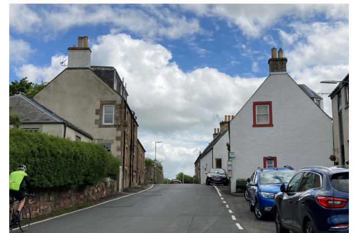
Fig. 26 (bottom): Gable ends are prominent in the conservation area. They tend to incorporate chimney stacks and some limited fenestration.
