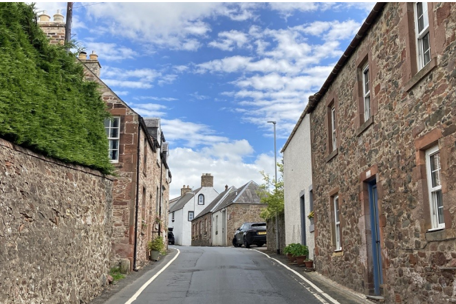
Fig. 15 Within the conservation area, the gentle curve of roads in the area create a series of unfolding views along their length. This creates an intimate atmosphere to the village.
